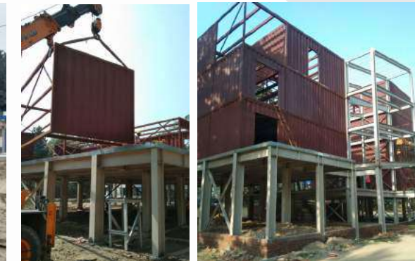
CONTAINER ERECTION
